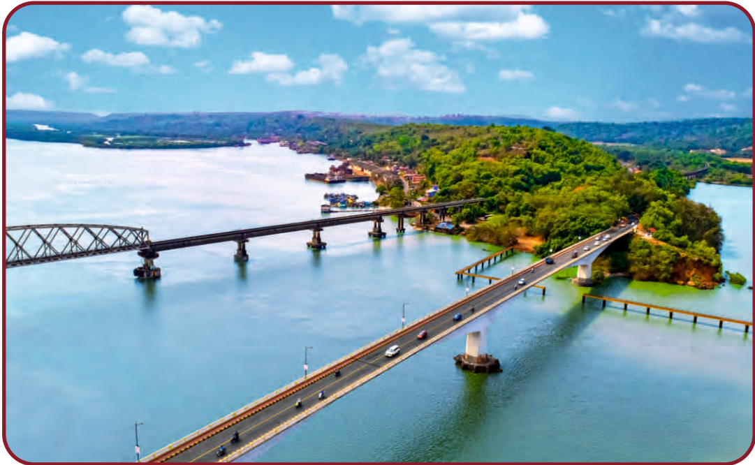
NH 66 Zuari Bridge, Goa
